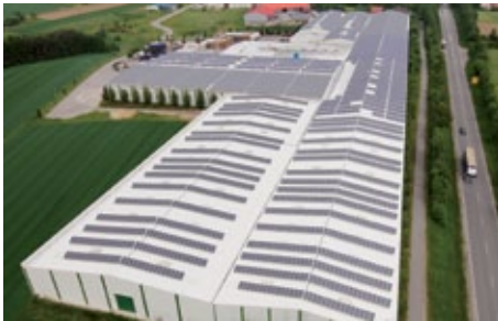
Simbach, Germany Plant capacity: 1 MW
